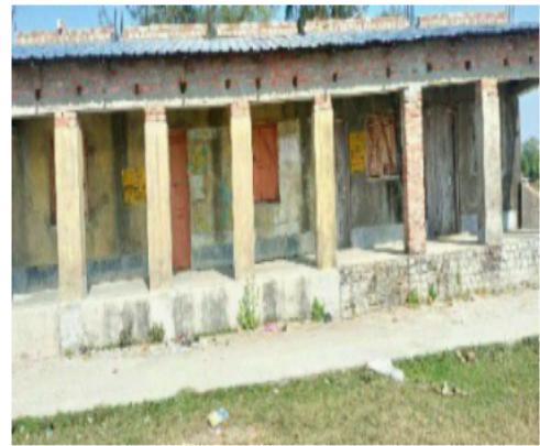
Polling Station Front View
