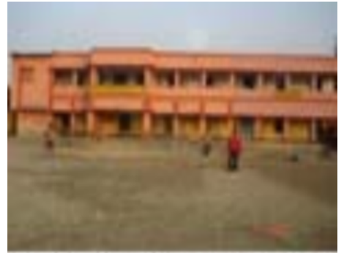
129(80) - Gopalnagar Tahala F.P. School (Room No. 1)
