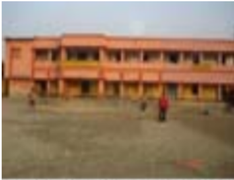
129(80) - Gopalnagar Tahala F.P. School (Room No. 1)
