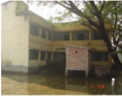
136/140 - Moydah F.P School (Room No. 2)
