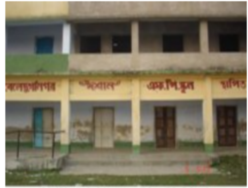
136/170 - Beledurganagar Ishan F.P. School
