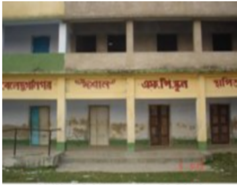
136/170 - Beledurganagar Ishan F.P. School
