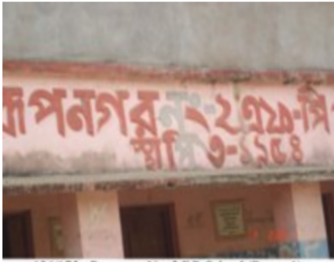
136/175 - Rupnagar No. 2 F.P. School (Room-1)
