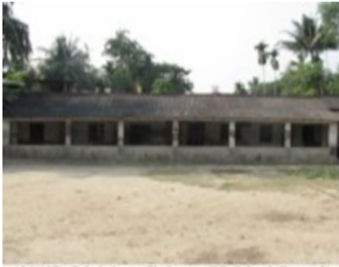
136/197 - Sahajadpur Chuknagar F.P. School (Room-2)
