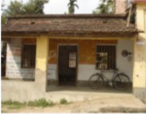
136/208 - Tulshighata F.P. School (Room No. 2)
