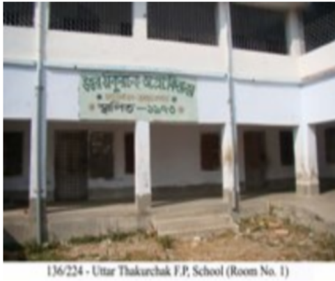
136/224 - Uttar Thakurachak F.P. School (Room No. 1)
