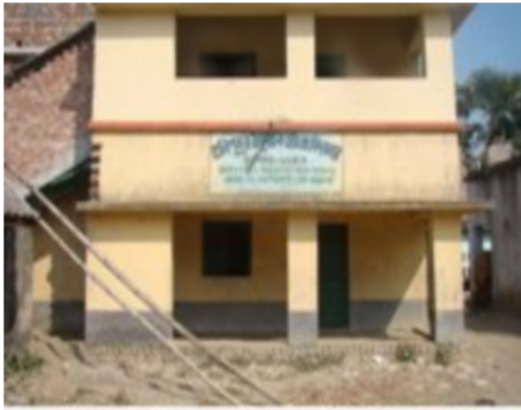
136/229 - Telepukur Thakurchak F.P. School (Room No. 1)
