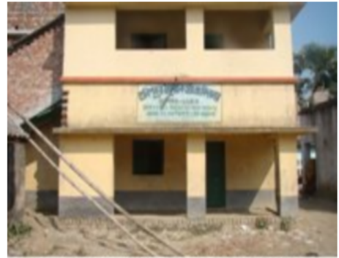
136/231 - Telepukur Thakurchak F.P. School (Room No. 3)
