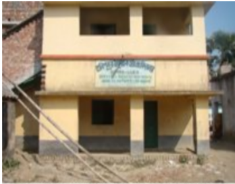
136/231 - Telepukur Thakurchak F.P. School (Room No. 3)
