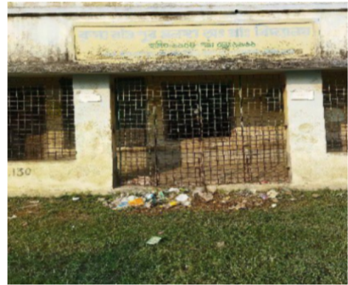
Polling Station Front View
