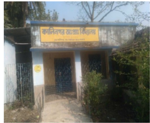
Polling Station Front View
