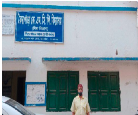
Polling Station Building Front View
