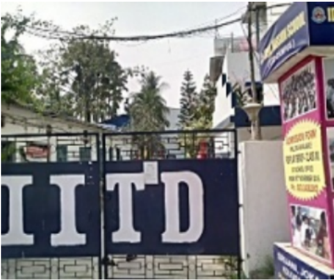
Polling Station Building Front View
