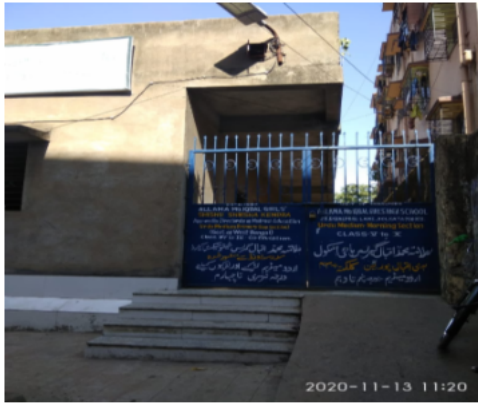
Polling Station Building Front View
