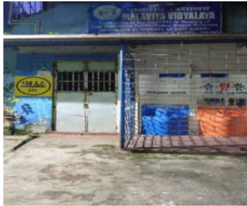
Polling Station Building Front View
