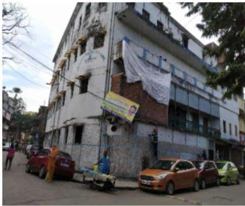
Polling Station Building Front View
