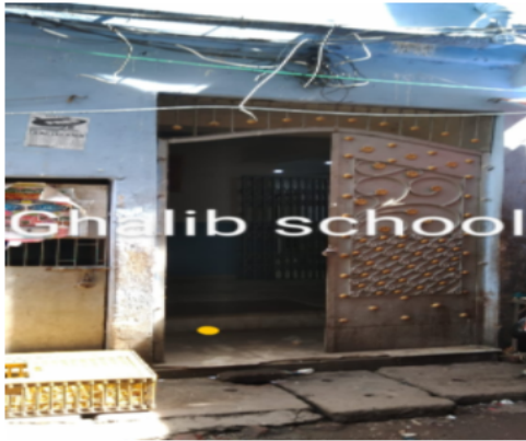
Polling Station Building Front View
