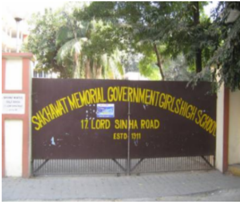
Polling Station Building Front View
