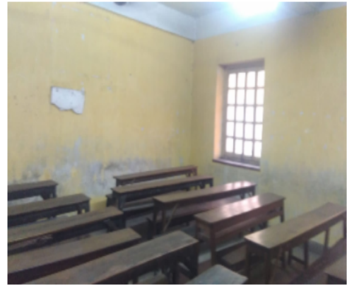
Polling Station Front View
