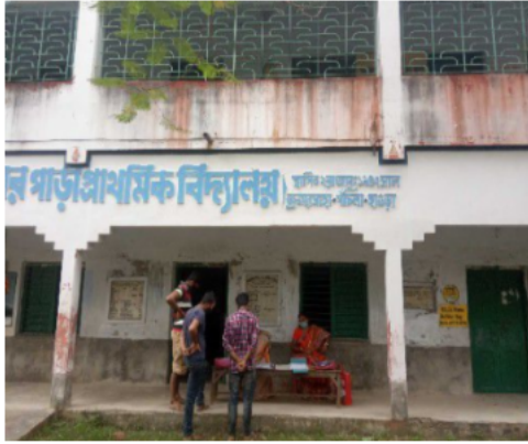
Polling Station Building Front View
