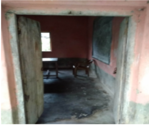
Polling Station Building Front View
