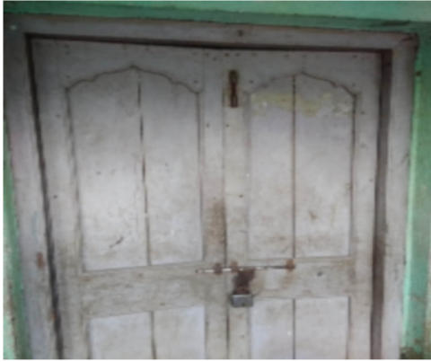
Polling Station Building Front View
