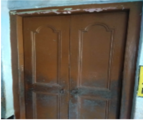
Polling Station Building Front View
