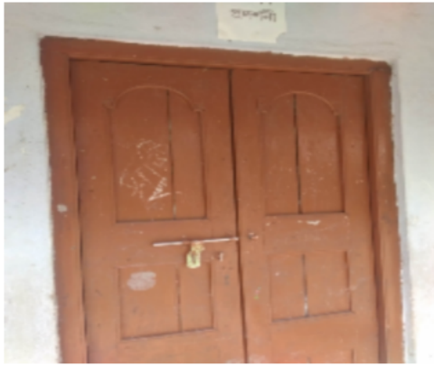
Polling Station Building Front View
