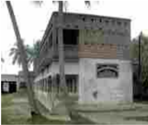
Polling Station Building Front View
