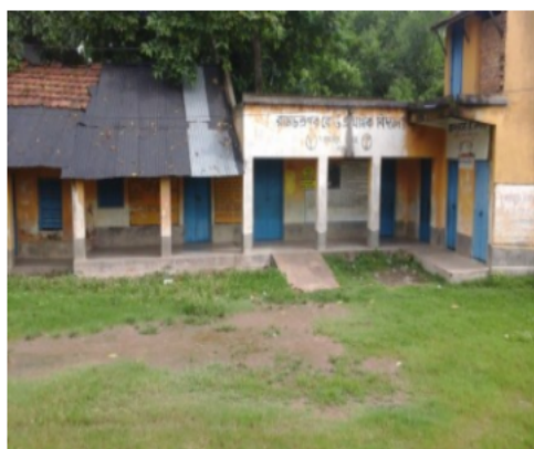
Polling Station Building Front View
