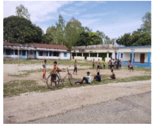
Polling Station Front View
