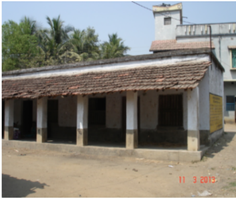
Polling Station Building Front View
