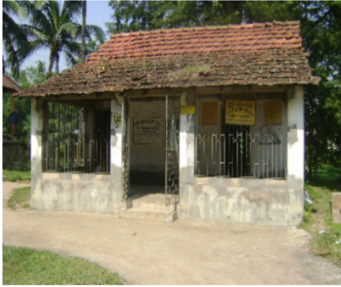
Polling Station Building Front View
