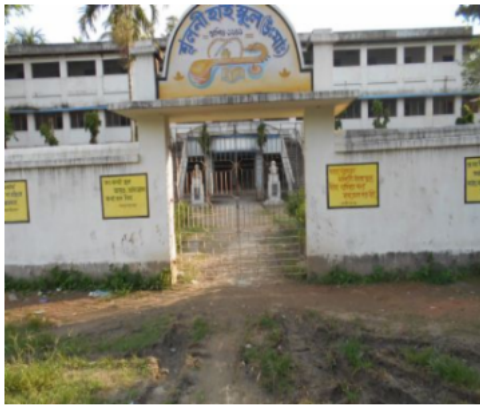
Polling Station Building Front View
