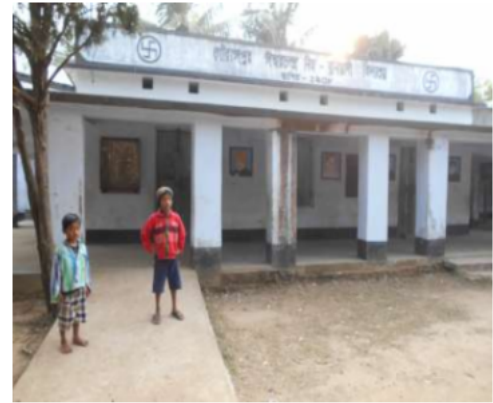
Polling Station Front View
