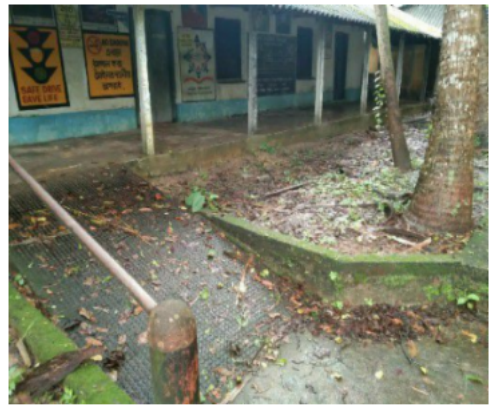
Polling Station Front View
