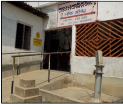
Polling Station Building Front View
