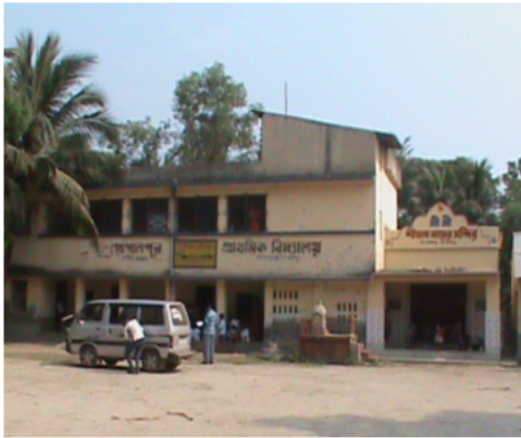
Polling Station Building Front View
