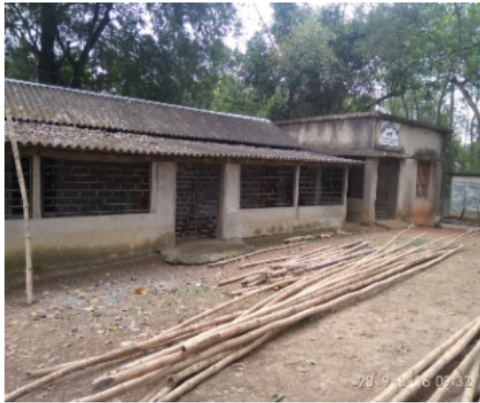
Polling Station Building Front View
