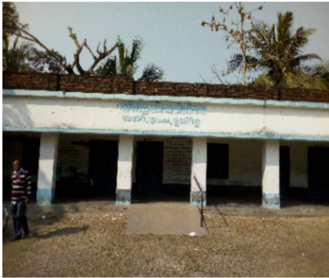
Polling Station Building Front View
