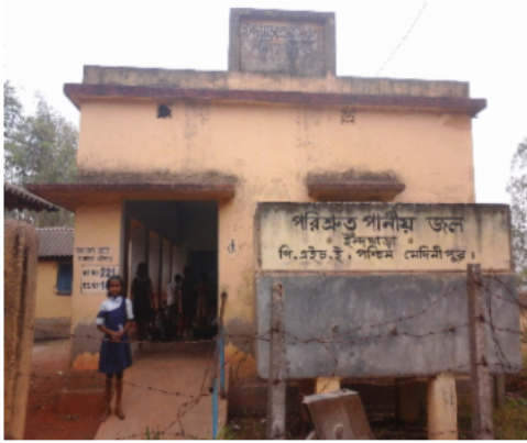
Polling Station Building Front View
