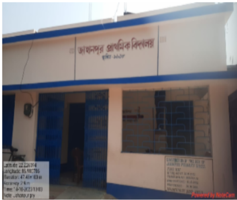
Polling Station Building Front View
