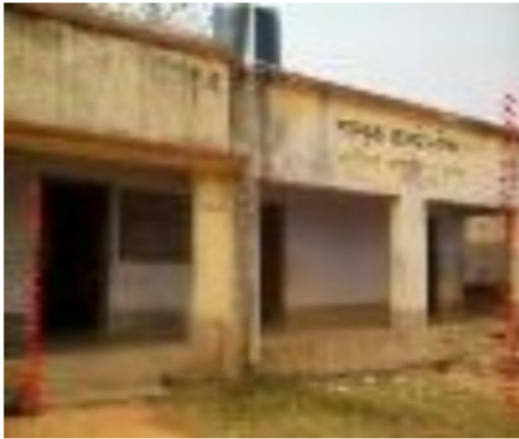
Polling Station Building Front View
