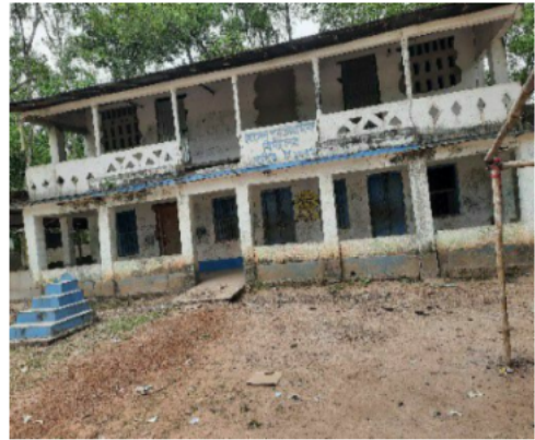
Polling Station Front View
