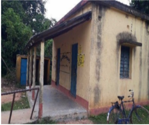
Polling Station Building Front View
