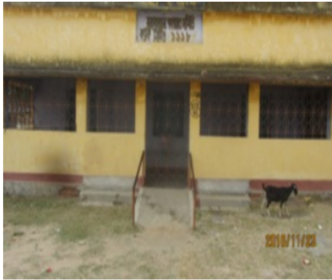
Polling Station Building Front View
