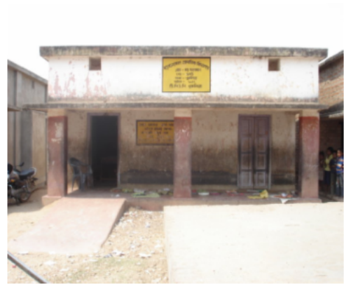
Polling Station Front View
