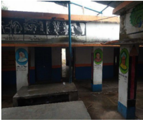
Polling Station Building Front View
