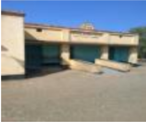
Polling Station Building Front View
