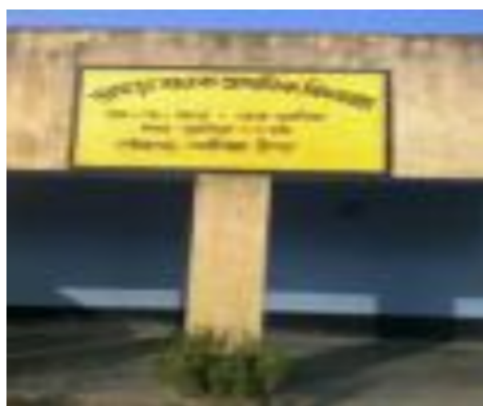
Polling Station Building Front View
