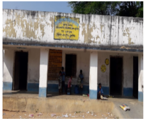
Polling Station Front View
