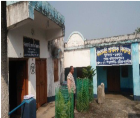
Polling Station Building Front View
