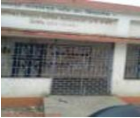
Polling Station Building Front View
